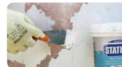
STEP 4: If there are bigger levelling needs, please apply STATUS ONE COVER .
