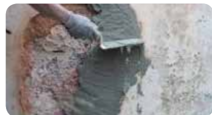
STEP 3: Apply fast setting WRM 520 on the surface of application. Wait 20 minutes to get dried.
