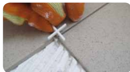
STEP 3: Distances between ceramic tiles can be easily fixed with the relevant special items (+, T, Y).
