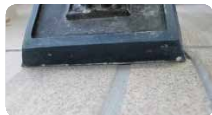
STEP 4: Apply FMF 150 tile grout at the desired tone.
