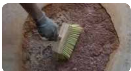
STEP 2: Prime the surface with the deep penetration primer GLX 292 FLEX PRIM .
