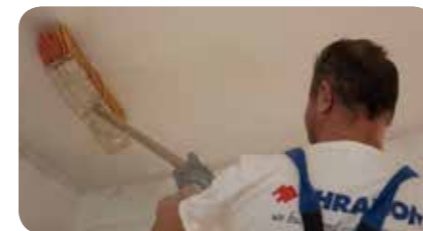
STEP 1: Thorough cleaning of surface from dust by using a metal brush.
