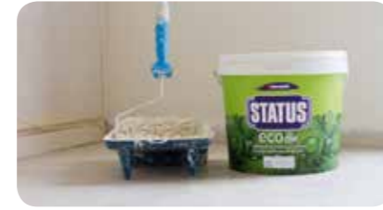
STEP 8: Apply STATUS ECO , ecological emulsion paint, in two coats.
