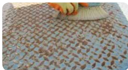
STEP 1: Thorough cleaning of surface from dust with a brush.
