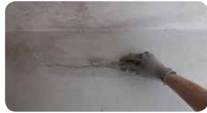
STEP 1: Widen the cracks and remove of dust and loose particles.
