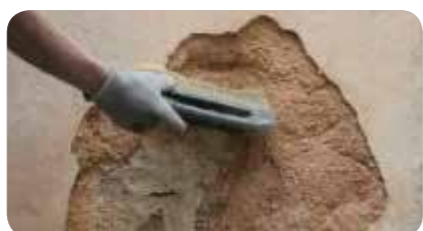
STEP 1: Remove crumbled plaster with a spatula and clean thoroughly the surface from dust.
