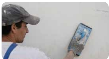
STEP 5: Once WRM 483 CEM COAT has dried, proceed to rubbing of surface.
