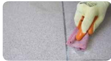
STEP 4: Good cleaning of surface with a wet cloth.
