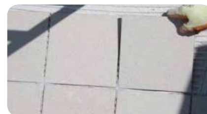
STEP 4: Distances between ceramic tiles can be easily fixed with the relevant special items (+, T, Y).
