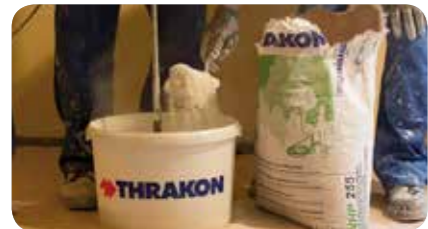
STEP 10: Apply NHP 250 one coat white plaster with marble.
