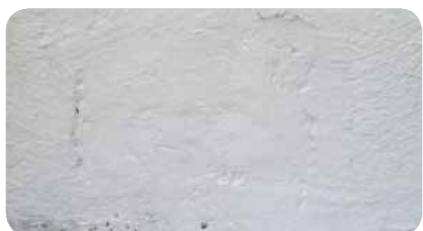
STEP 7: Paint the surface with STATUS ALL WEATHER in two layers.
