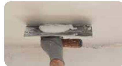
STEP 12: In case finer surface is required, use the DEC 470 FINE putty.
