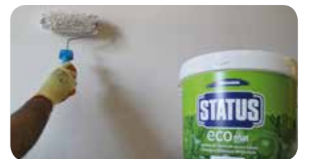
STEP 6: Apply STATUS ECO , ecological emulsion paint in two coats.
