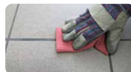
STEP 4: After tile grout has dried, clean the surface with a sponge.
