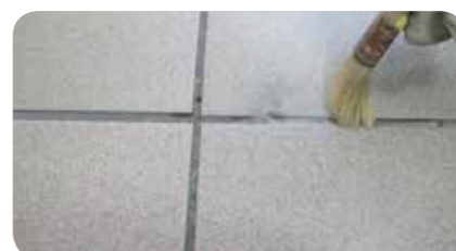
STEP 2: Clean thoroughly the surface from dust. Light cleaning with water is suggested.
