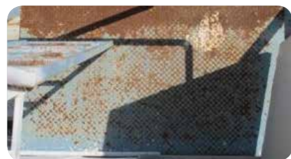
In these cases apply VKW 132, as long as the application is not bigger than 5 m 2 .
