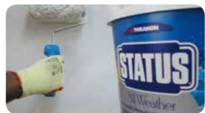
STEP 9: Apply STATUS ALL WEATHER in two layers.
