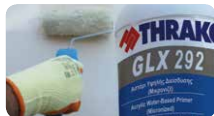
STEP 6: Apply deep penetration primer, GLX 292 FLEX PRIM .
