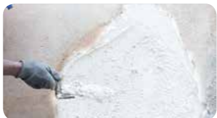
STEP 4: Apply WRM 483 CEM COAT which is a cementitious putty.
