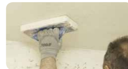
STEP 4: After 10 - 12 hours, rub the surface with a wet sponged trowel for making the surface smoother.
