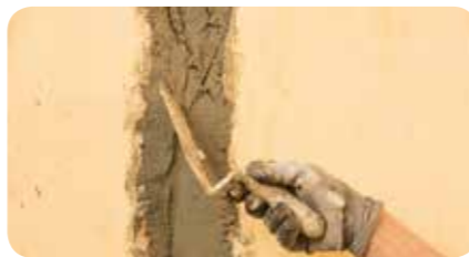
STEP 3: Before WRM 518 starts getting dry, engrave it diagonally for increased bonding and easier application.
