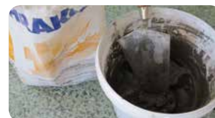
STEP 3: The mix is prepared, having chosen one of THRAKON's FMF 160 tile grouts and applied with a rubber spatula.
