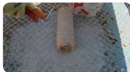
STEP 2: Apply the GLX 190, quartz sand primer, for increased bonding.
