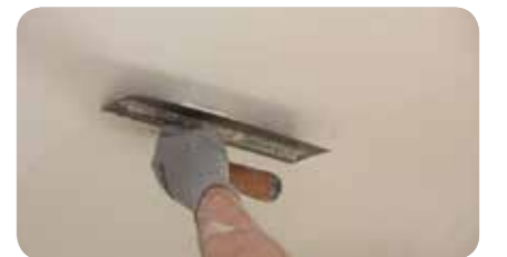
STEP 3: Apply DEC 470 , with a spatula, in two coats.
