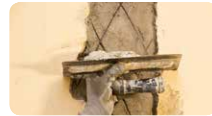
STEP 4: Apply WRM 483 CEM COAT FINE , an extra-fine cementitious putty.
