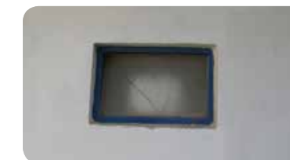
STEP 5: Application of STATUS ALL WEATHER in two layers.
