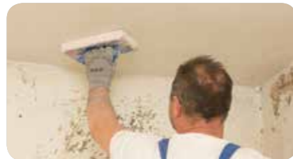
STEP 11: Rub the surface with a sponged trowel.
