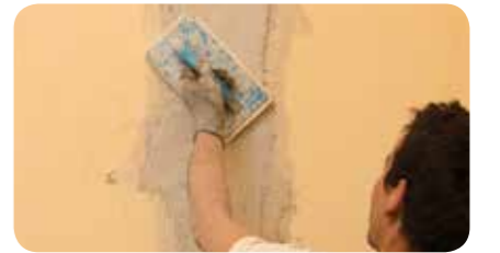
STEP 6: Leave WRM 483 CEM COAT FINE to get dried and rub with a wet sponged trowel for making the surface smoother.
