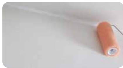
STEP 5: Apply GLX 292 FLEX PRIM , deep penetration primer.
