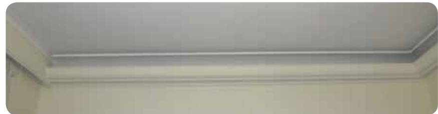
STEP 10: Apply NHP 250 one coat white plaster with marble.
