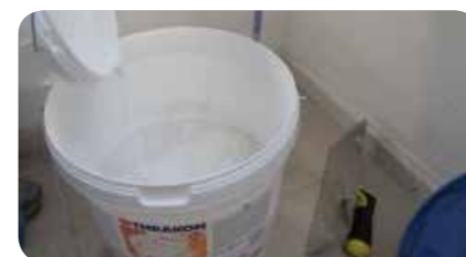
STEP 3: Apply the elastic tile adhesive, VKW 132. It is a two component product, ideal for applications under contractions and expansions.
