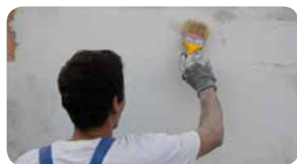
STEP 8: Prime the surface with STATUS DUR , solvent based primer.
