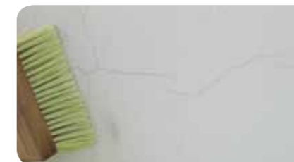
STEP 1: Clean thoroughly the surface from dust and loose particles, with a brush.
