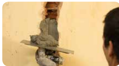
STEP 2: Filling of gap should be done with fast setting repairing product WRM 518 (R2).
