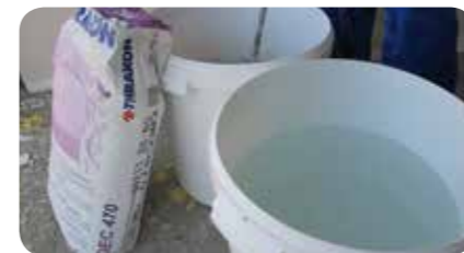
STEP 2: Preparation of mixture by placing the required amount of DEC 470 in a clean bucket. Then add water gradually, while you stir the content of the bucket.
