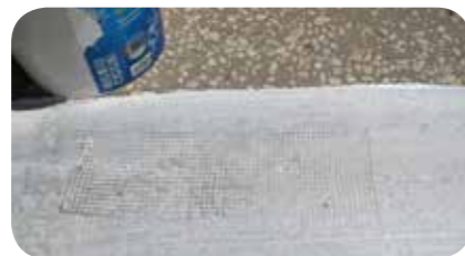
STEP 4: While the first layer is still wet, apply a strip of THRAKON fiberglass tape along the joint.
