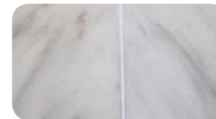
STEP 4: Apply silicone SEAL POOL , which is ideal for applications with moisture and intense contractions.
