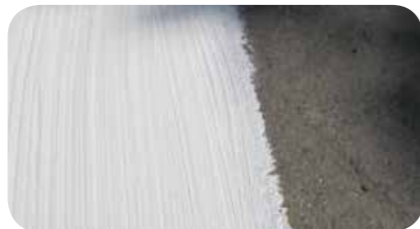
STEP 4: Cut the THRAKON fiberglass tape to the dimensions needed so as to cover the crack fully.
