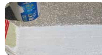
STEP 6: After the first layer of FLX 380 ROOF SEALER has dried, a second layer is applied along the joint.
