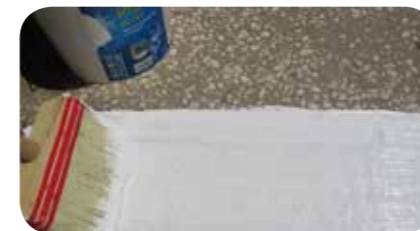
STEP 5: Press the tape in order to enforce FLX 380 ROOF SEALER .
