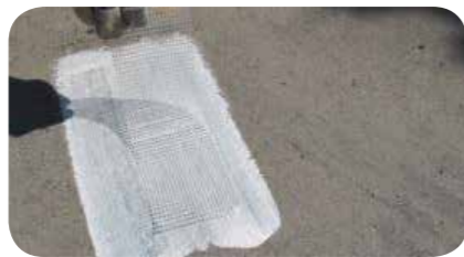
STEP 4: Cut the THRAKON fiberglass tape to the dimensions needed so as to cover the crack fully.
