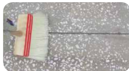
STEP 1: Clean the surface thoroughly from loose particles and dirt.
