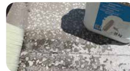
STEP 2: Prime the surface with the deep penetration primer, GLX 292 FLEX PRIM .
