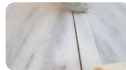
STEP 3: Apply paper tape on the left and right sides of the joint in order to avoid dirtying the surface.
