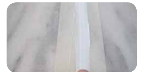
STEP 5: Flatten the surface with your finger, while SEAL POOL is still wet.
