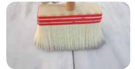
STEP 2: Clean the surface thoroughly from loose particles and dirt with a brush.
