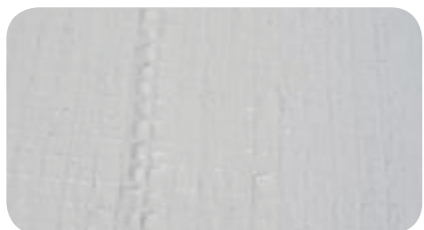
STEP 3: Apply the first layer of FLX 380 ROOF SEALER with a brush or a roll.
