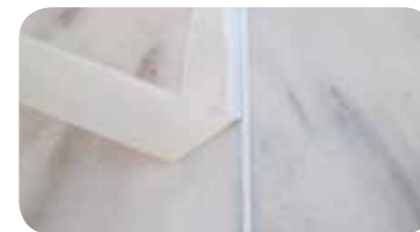
STEP 6: Remove the paper tape, while silicone is still fresh.
