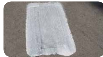
STEP 5: Apply the mesh over the crack by pressing it on its surface, while FLX 382 PLUS is still wet.
