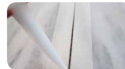
STEP 4: Apply silicone SEAL POOL , which is ideal for applications with moisture and intense contractions.
