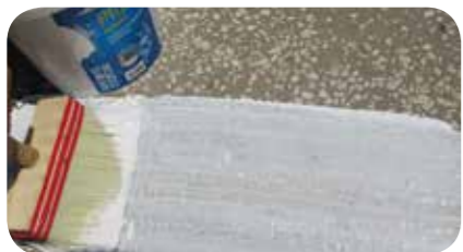
STEP 3: Apply the first layer of FLX 380 ROOF SEALER with a brush or a roll.
