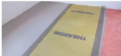
Fiberglass mesh to be applied next to each other, overlaying by 10cm
