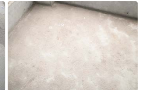
Surface ready for application
