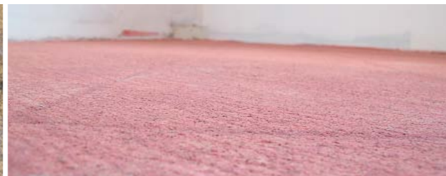
Floor priming (Quartz primer)
