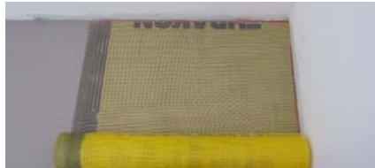
The application starts from the corner of the room
