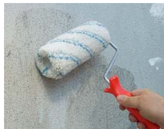
Masonry priming
