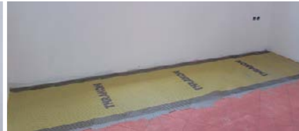
Apply fiberglass mesh throughout the length
