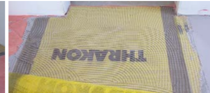
Cut the fiberglass mesh for shaping on doors
