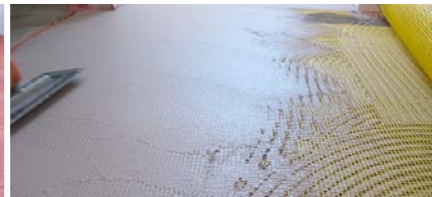
Along the way we use the smooth trowel to level the surface
