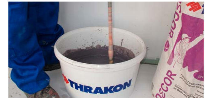
DECOR Mixture preparation
