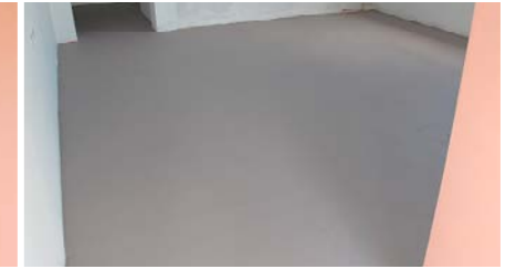
Where necessary we apply more layers, with smooth stainless steel trowel.
